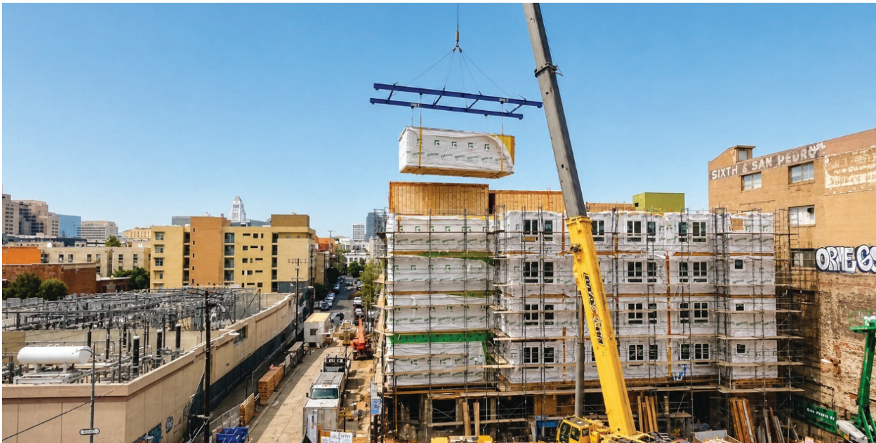
FIGURE 3 | Full modular construction – Mercy Housing (LA, California)
